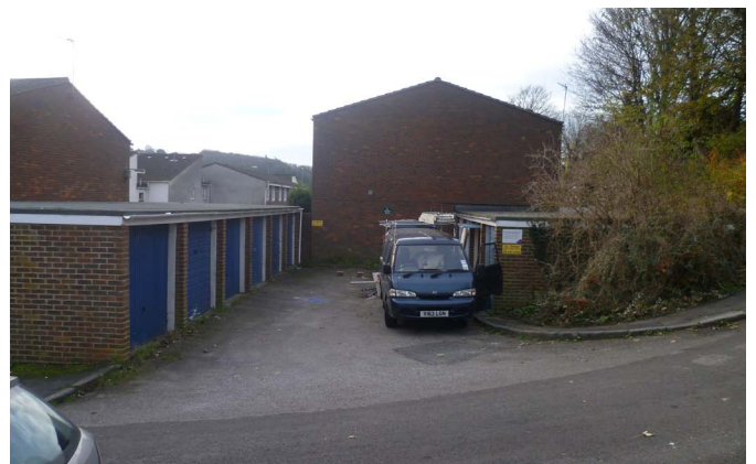
View looking South into the Site
